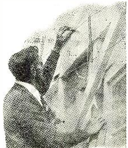
Norman McConnell, operating at Pylon No. 2, is shown at the left. At the right, Al H. Gyssler (W8BXB) is using a neon tube to find the nodal point on the antenna system at the headquarters station
